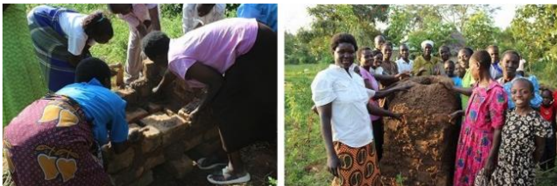
A workshop held by Takuro on how to build an oven suited for making charcoal
